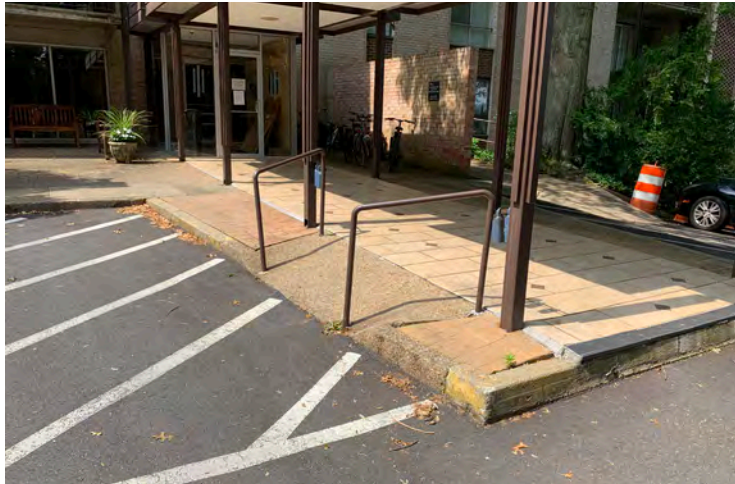
CURB RAMP IN NOT ADA-COMPLIANT
