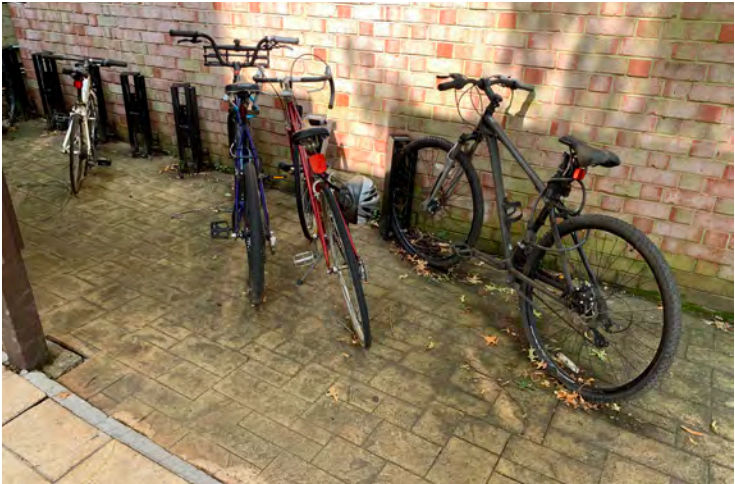
CERAMIC TILES ARE SLIP HAZARDS; BEVELED EDGES ARE NOT ADA-COMPLIANT; PAVING AT BASE OF CANOPY POST FAILING
