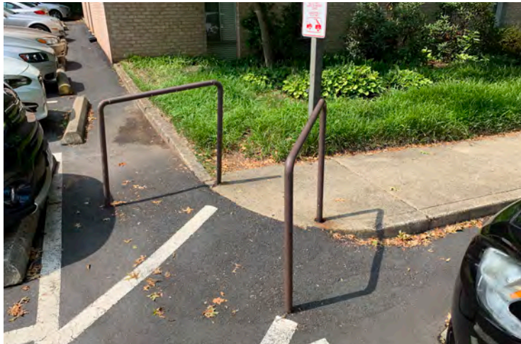
CURB RAMP IN NOT ADA-COMPLIANT
