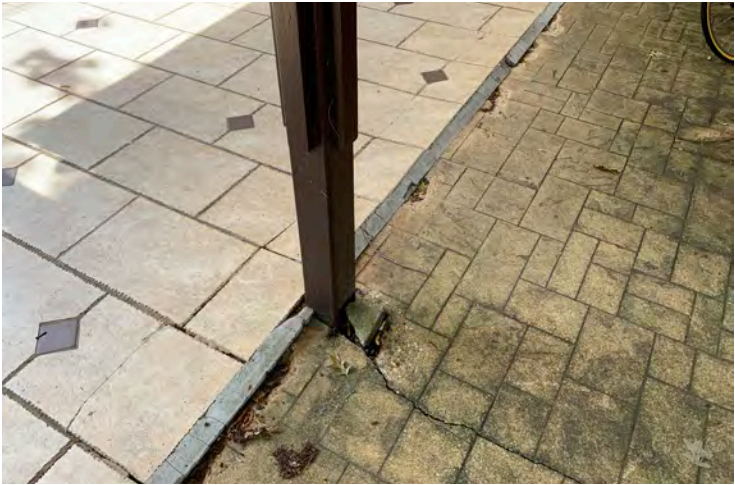
CERAMIC TILES ARE SLIP HAZARDS; BEVELED EDGES ARE NOT ADA-COMPLIANT; PAVING AT BASE OF CANOPY POST FAILING
